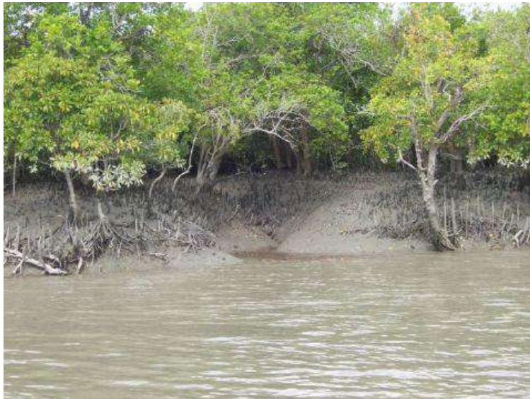
Mangrove root system beginning to erode along the Sundarban coast.
